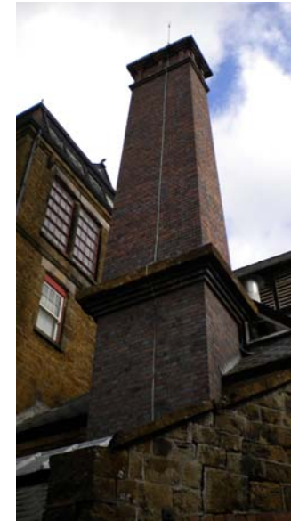
Hook Norton Brewery - Chimney repairs.
