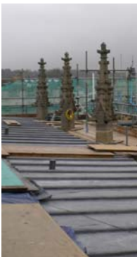
St Mary the Virgin Church High Street, Oxford Roof works.
