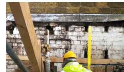
Hook Norton Brewery - Roof repairs.
